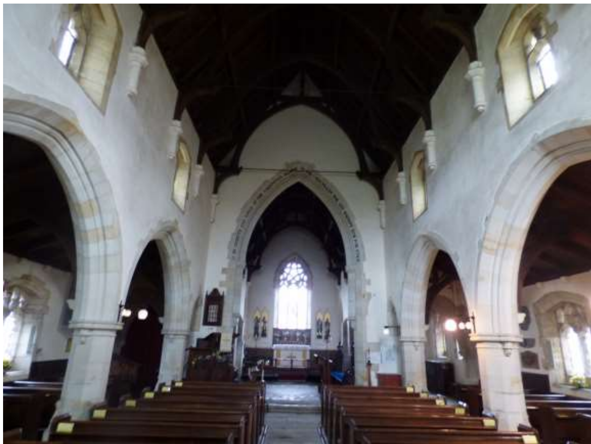
17. General view of nave looking east.
