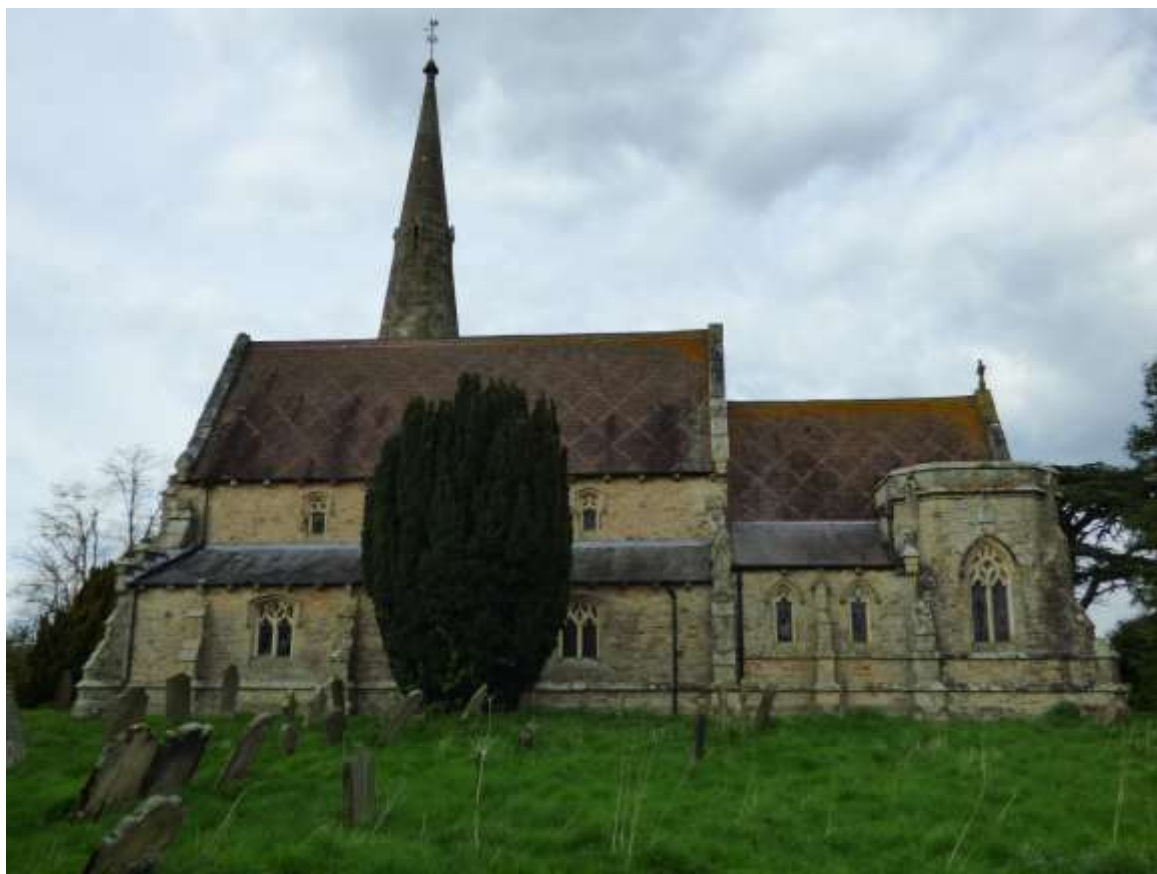
1. General view of south side of church.
