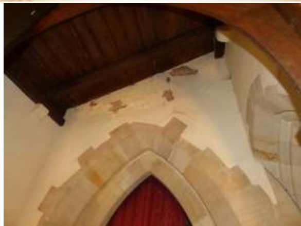
20. Damp ingress to underside of roofs, clockwise from top left: south side of porch; toilet; east end of north aisle; west end of south aisle.
