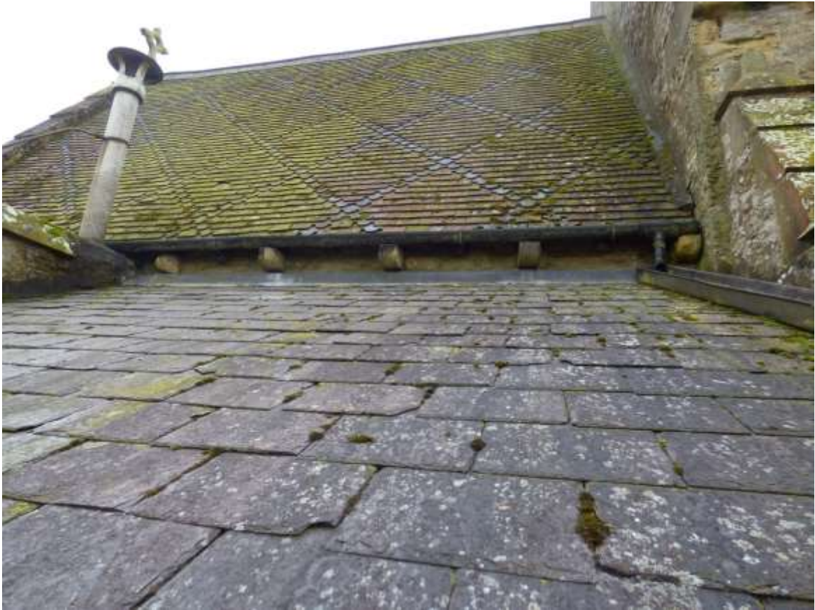
14. General view of vestry roof.
