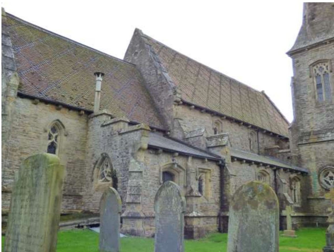
3. General view of north side of church.
