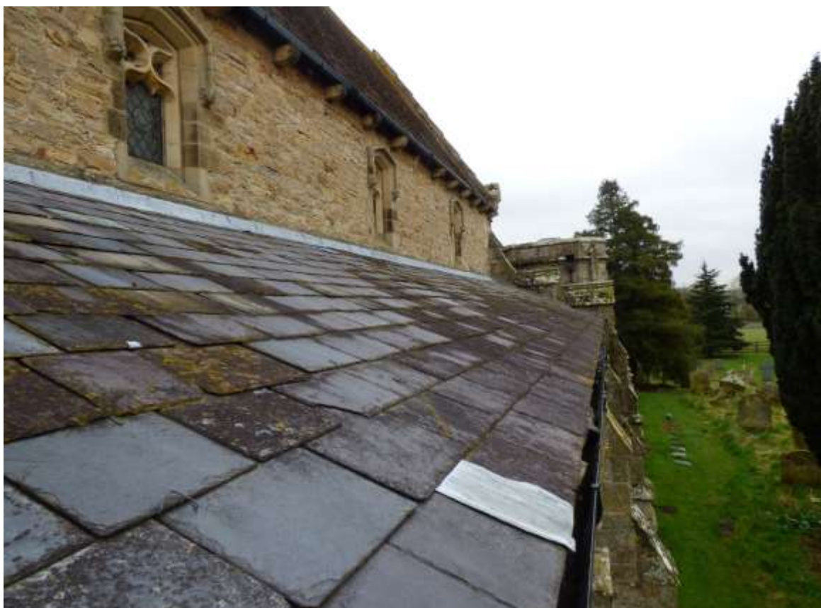
13. General view of south aisle roof.
