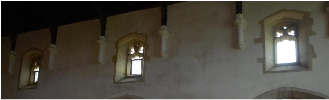
South aisle clerestory SII SIII SIV
