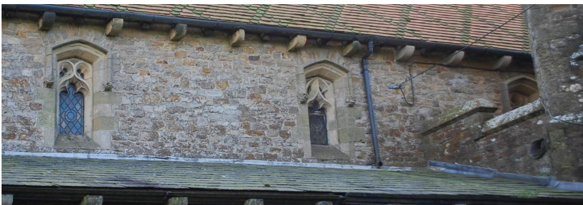
North aisle clerestory from exterior NII NIII NIV
