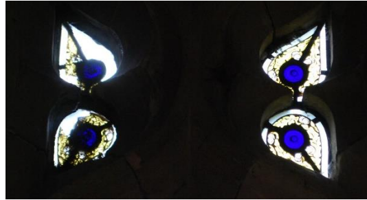
Detail, damage and loss to left-most tracery
