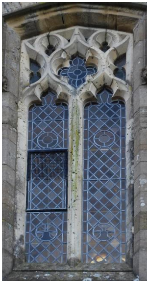
Tower, East Window
