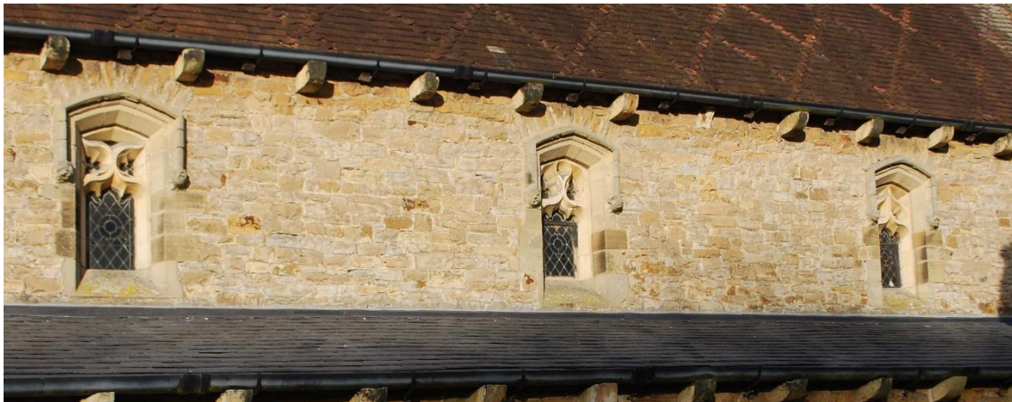
South aisle clerestory from exterior SIV SIII SII
