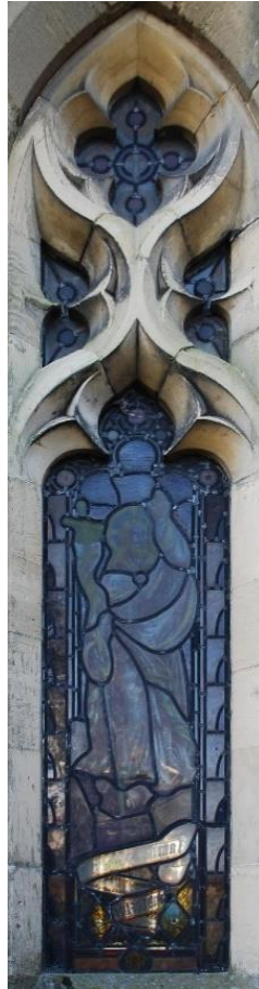
Detail, damage and loss to left-most tracery
